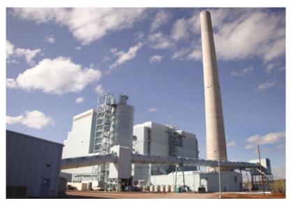
The 420MW-rated coal-fired unit at Basin Electric's Dry Fork Station has operated the world's largest CFBS since it entered service in June 2011. Since it began operation, the CFBS has exceeded its design performance reducing SO<sub>2</sub> by 95 percent to 98 percent. Photo Courtesy: Basin Electric Co-Op and Wyoming Municipal Power Agency
