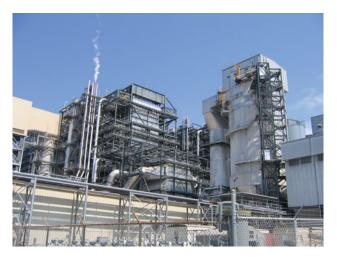
JEA's Northside Generating Station includes two Amec Foster Wheeler CFB boilers, each producing 831,000 ACFM of flue gas. Each boiler uses a single SDA followed by a pulse jet fabric filter to treat the flue gas produced by the pet coke- and coal-fired unit. SO<sub>2</sub> emissions are reduced up to 90 percent and SO<sub>3</sub>, HCl, and HF emissions are reduced up to 99 percent. The plant has been in operation since 2002. Photo Courtesy: Amec Foster Wheeler
