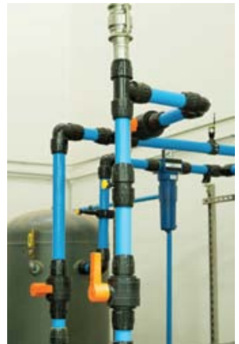
Figure 2. Transair aluminium piping uses Quick-Connect connections
