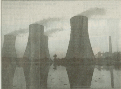
Cooling towers stand at the NTPC Ltd. power station in Dadri, India, earlier this month. Krishnan & Associates of Stamford is working with the Indian industry to increase power capacity and the capabilities of its personnel.
