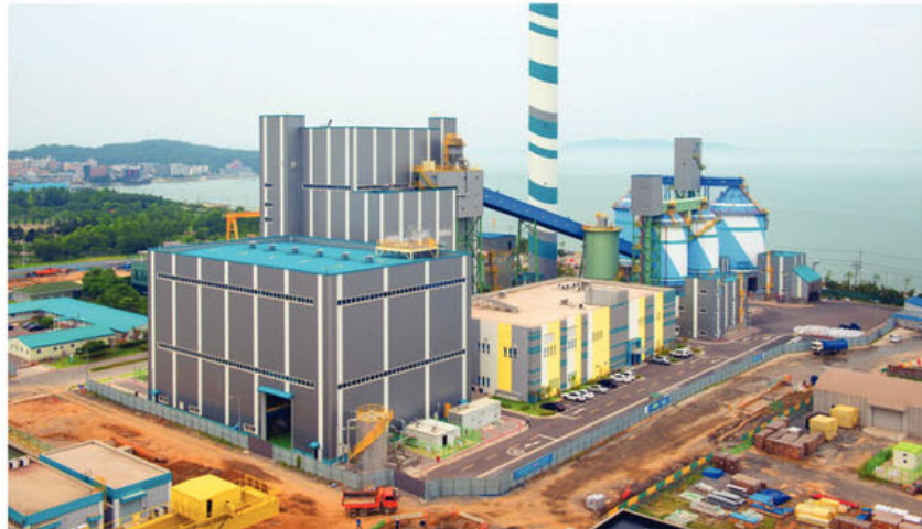
1. GS Electric Power and Services' 105-MW Bio-1 circulating fluidized bed (CFB) plant in Dangjin, South Korea, is the largest biomass-fired power plant in Asia. Courtesy: Sumitomo SHI FW (SFW)
