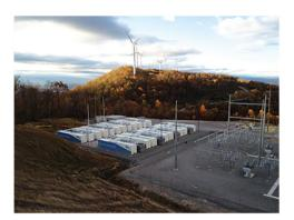
The 98MW Laurel Mountain Wind Farm uses battery energy storage to optimize energy sold into PJM and to provide regulation services.
