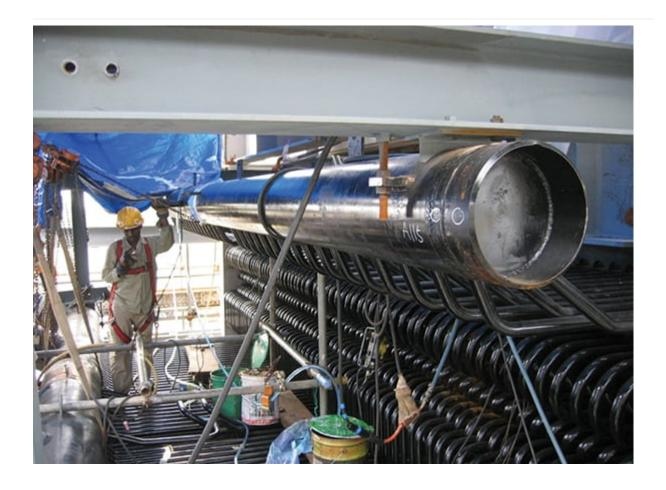
**3. Minimize field welds.** Once a module is lifted into place and secured, the single inlet and outlet headers are welded together. Note the absence of "jumper pipes" and headers common on horizontal HRSGs. The elbows were shop welded and the complete module hydro tested before leaving the factory. *Courtesy: CMI Energy*
