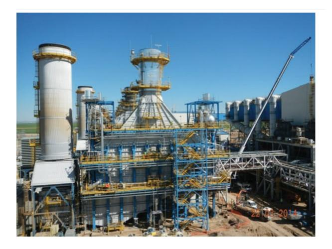
**5. Flexible operations.** One of the eight HRSGs is shown with the CT on the far left, with the diverter damper and bypass stack shown between the CT and the HRSG. The diverter damper allows operation of the CTs in simple cycle mode by bypassing the CT's exhaust gases before entering the HRSG. *Courtesy: CMI Energy*
