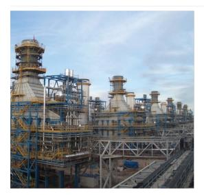
**1. Phased construction.** The Erbil Gas Power Station was constructed in three phases. The first and second phases each consisted of four GE Frame 9E combustion turbines (CTs). Phase 3 added eight CMI Energy heat-recovery steam generators (HRSGs) and two GE steam turbines, forming two 4 x 1 power blocks. The plant, rated at approximately 1,500 MW in combined cycle mode, is the largest power plant in Iraqi Kurdistan. *Courtesy: CMI Energy*
