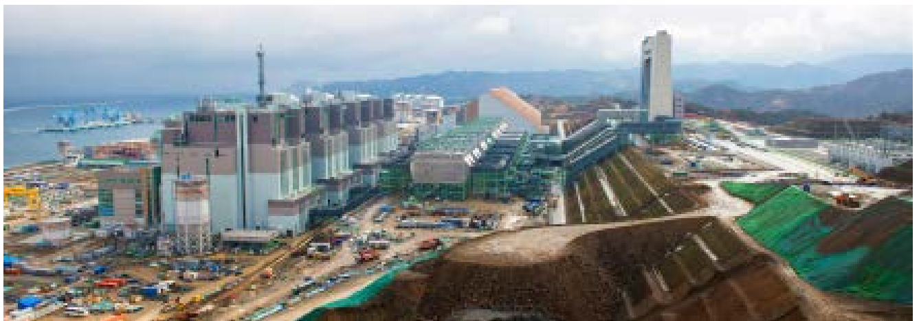
Figure 6. The 2200 MWe Green Power CFB plant in Samcheok, South Korea. Source: Sumitomo SHI FW
