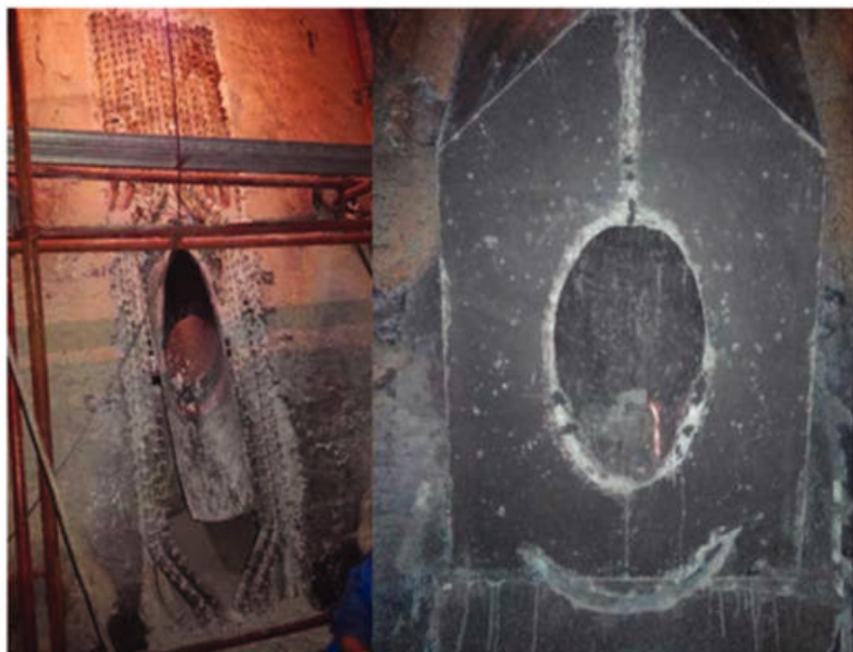
3. Fuel chutes before (left) and after (right) SFW's refractory lining upgrade shows elimination of radiation damage. Courtesy: Sumitomo SFW
