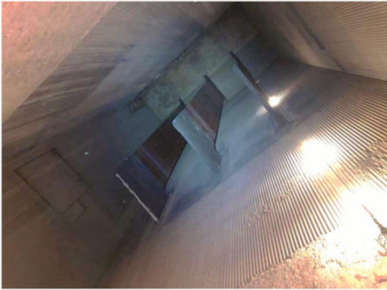
2. Typical wingwall evaporative surface. Courtesy: Sumitomo SFW
